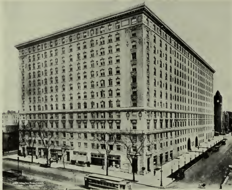
BELNORD APARTMENT BUILDING, BROADWAY, NEW YORK CITY. Exterior and courts of light gray Kittanning brick, furnished by Pfortenhauer-Nesbit Company. Hiss & Weeks, Architects.
